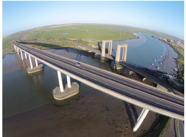
Figure 1 New Sheppey Crossing
