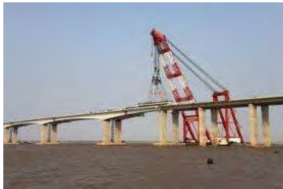
Figure 4: Sheer leg for erection of moving span
